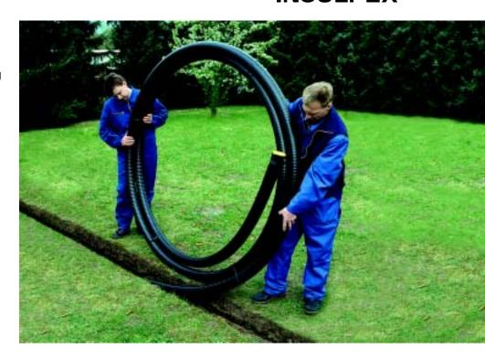
INSULPEX has a long life expectancy at typical operating temperatures and pressures. It does not corrode and is resistant to aggressive soil and water.
